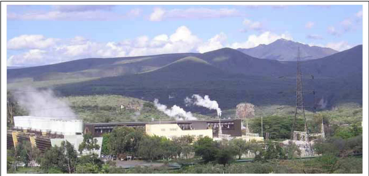
Geothermie – Kraftwerk in Olkaria, Kenia. © KfW
