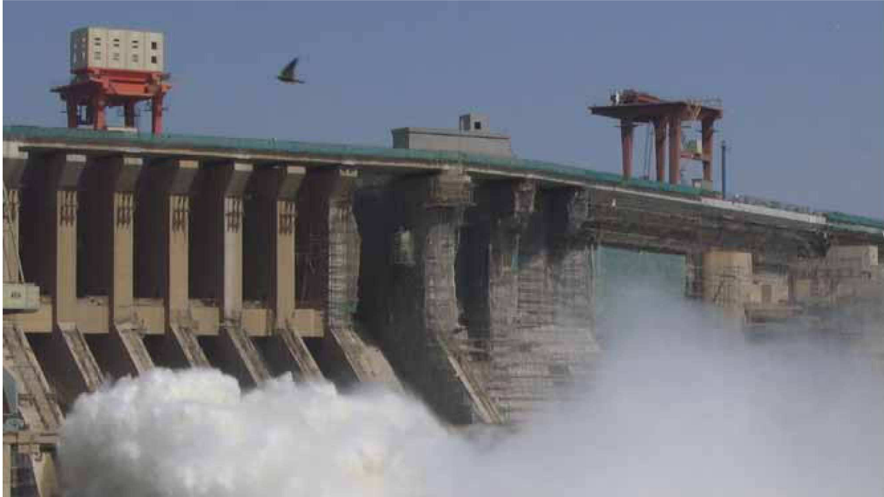
Merowe Dam in Northern Sudan © GIZ
